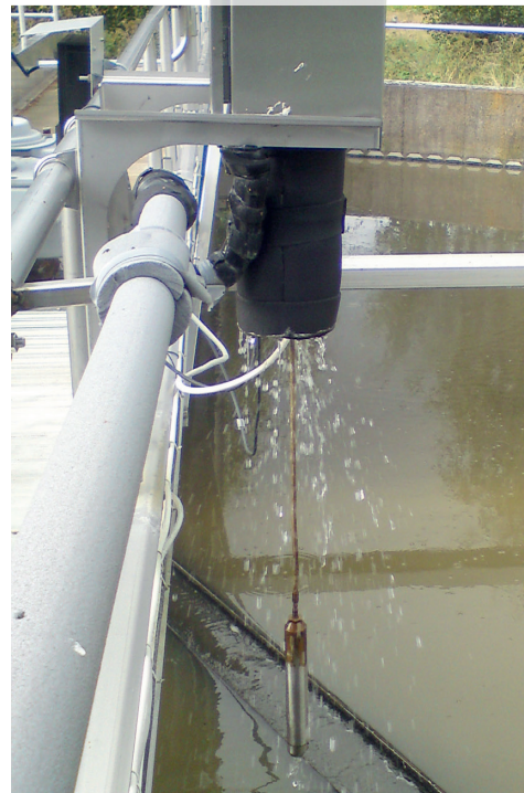
The CBX is built into a stainless steel enclosure for installation in a variety of environments. It has automatic flushing of both sensor and cable after each sampling.
