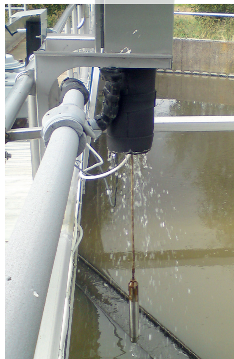
The CBX is built into a stainless steel enclosure for installation in a variety of environments. It has automatic flushing of both sensor and cable after each sampling.
